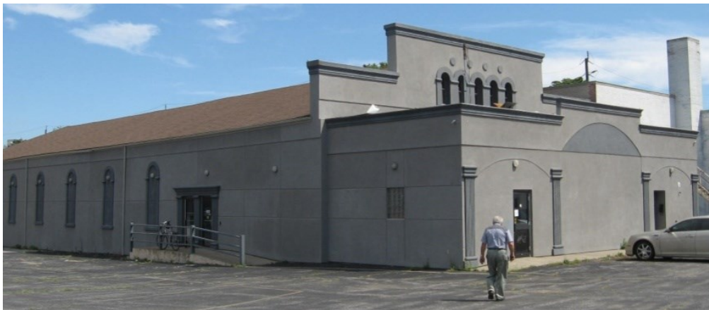
Photograph of the east barn building, dated July 2012, showing the south addition and grey painted stucco, with parapet and arched windows visible from the street
