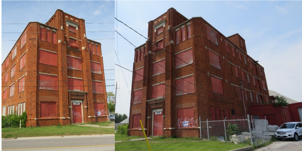
Front views of 10150 Riverside Drive East
