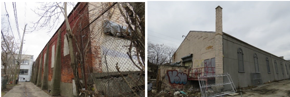
Photographs of the east barn building, showing the alley-facing east wall, concrete buttresses, and painted brick on the north face
