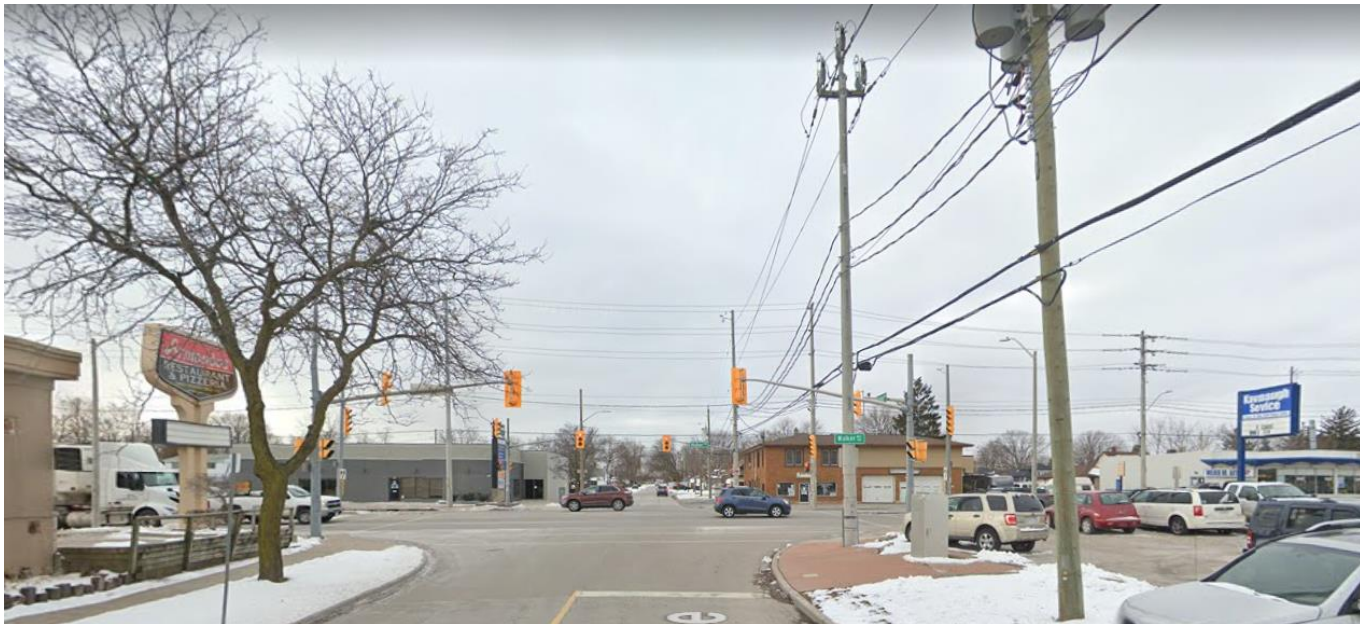
View of Walker & Sydney intersection looking east from west side of Walker (near Turner Rd) 8
